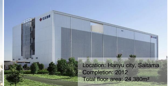
The Sumitomo Warehouse Hanyu Archives Center 2
