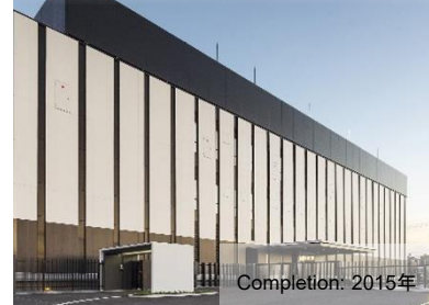
QTnet Service Operations Center
