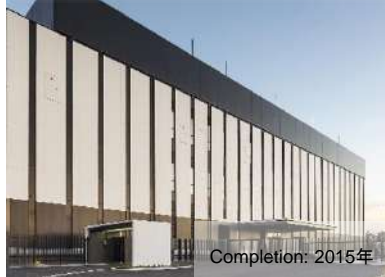
QTnet Service Operations Center*
