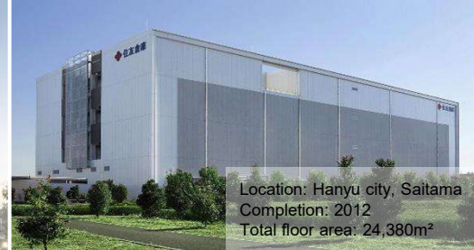
The Sumitomo Warehouse Hanyu Archives Center 2*
