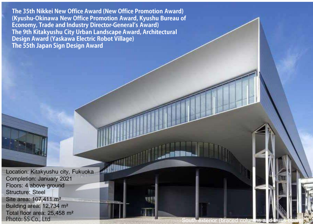
South exterior (braced columns and truss beams)
